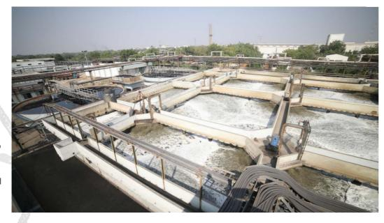
Arvind Envisol has designed the state-of-the-art Sewage Treatment Plant (STP) plant based on analysis of composite samplings at pumping stations. The water is treated and further polished at our STP through various technologies such as bar screening, pH correction, flash mixer, primary clarifier and sand filter.
